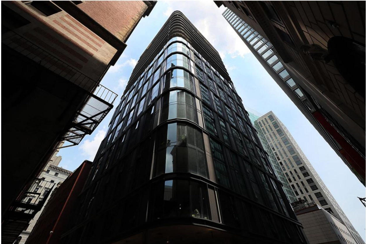
The Parker under construction on Lagrange Street in Boston. SUZANNE KREITER/GLOBE STAFF
