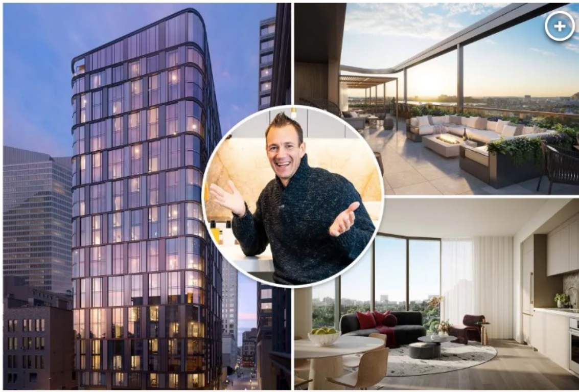
Gym dandy: Gronk (center) is designing slick residential fitness centers like this one in Boston's Parker building. The Parker
